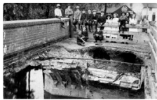
Picture of the collapsed section of the Old Bridge in 1912.
