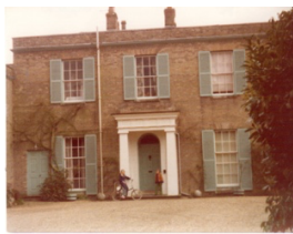
Picture of the front of the Old Rectory
